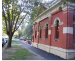
h00675 former gas valve house st kilda road st kilda along street she project 2004
