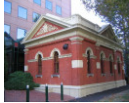
h00675 1 former gas valve house st kilda road st kilda street view she project 2004
