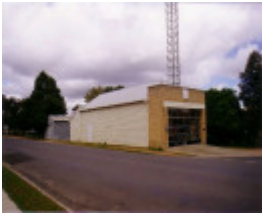
SD 258 - St. Arnaud Fire Station, Walker Street (corner Dundas Street), ST ARNAUD
