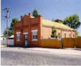
SD 265 - Former St. Arnaud Power House, Wills Street, ST ARNAUD
