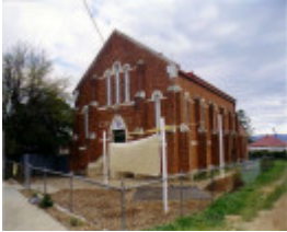
SL 002a - Stawell Scout Hall (former St. Mark's Presbyterian Church), 20 Alfred Street, STAWELL
