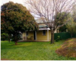
SL 006 - House, 1 Ann Street, STAWELL
