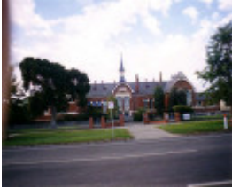
SL 008 - Stawell State School No 502, Barnes Street, STAWELL
