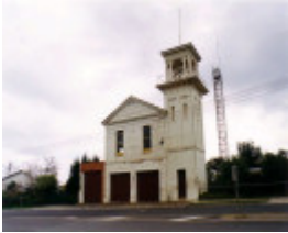
SL 024 - Former Stawell Volunteer Fire Brigade Station, 1 Byrne St , STAWELL
