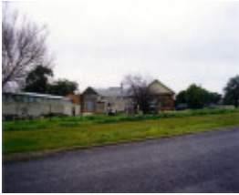
SL 069 - Former Stawell Butter Factory and Ice Company
