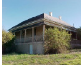
Ledcourt Exterior View May 2001
