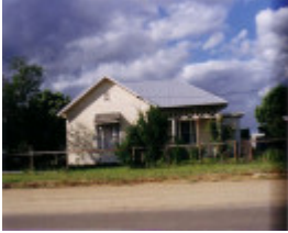
SL 135 - Former Telegraph Office, 21 Leslie Street, STAWELL
