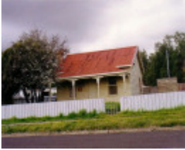
SL 151 - House, 6 Lillian Street, STAWELL
