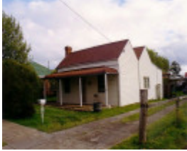
SL 152 - House, 7 Lillian Street, STAWELL
