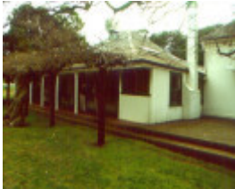
1 killeen homestead with verandah august2000.jpg
