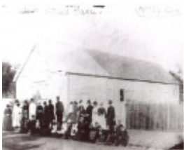
SL 183d - Barracks in Main St., Stawell Historical Society.
