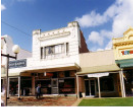
SL 197 - Two-storey Commercial Building
