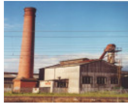
B6541 Former Australian Plaster Industries Boiler House
