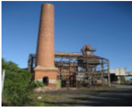
B6541 Former Australian Plaster Industries Boiler House
