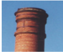
B6541 Former Australian Plaster Industries Chimney top
