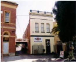
SL 229 - Two-storey building (part of former Commercial Hotel),
