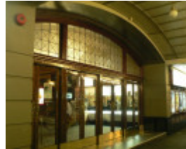
Regent Theatre Ballarat detail of entrance 2009
