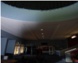
Midland Theatre Ararat foyer showing circular opening 2009
