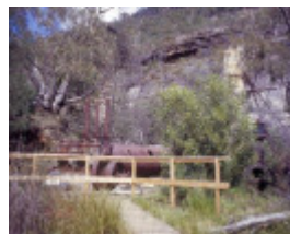
h01556 heatherlie quarry grampians national park halls gapp boilers chimney compressor she project 2004
