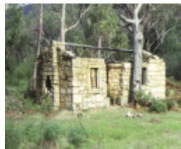
1 heatherlie quarry roses gap stawell building shell
