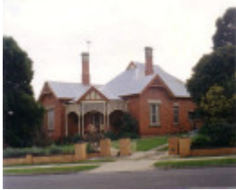
SL 279 - Former Presbyterian Manse, 9 Scallan Street, STAWELL
