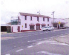
SL 290 - Former Stawell Coach Factory building (now 'Sniff N Tell'), Scotland Place, STAWELL
