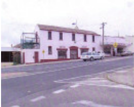
SL 290 - Former Stawell Coach Factory building (now 'Sniff N Tell'), Scotland Place, STAWELL
