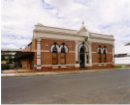
SL 333 - Jacaranda Restaurant at Stawell Technical School (former School of Mines)
