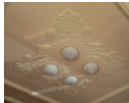
Horsham Theatre detail of ceiling 2009
