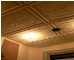
Horsham Theatre detail of auditorium ceiling 2009
