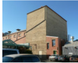
Horsham Theatre rear view of fly tower 2009
