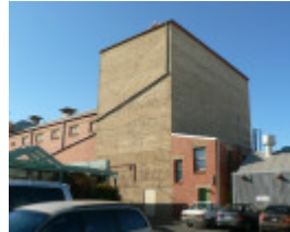
Horsham Theatre rear view of fly tower 2009
