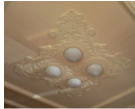
Horsham Theatre detail of ceiling 2009
