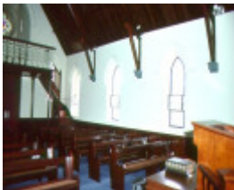
St Johns Streatham Interior September 2000
