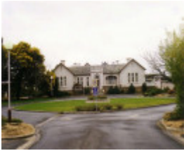
SL 413 - Pleasant Creek Hospital, Western Highway, STAWELL
