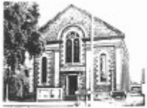
Uniting Church, 61 Percy Street, Portland, Glenelg Shire, 1982. No. 11 Percy Street.
