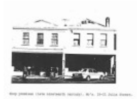
Shop Premises, 19-21 Julia Street
