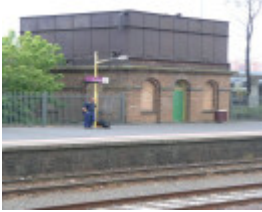
WATER TOWER SOHE 2008
