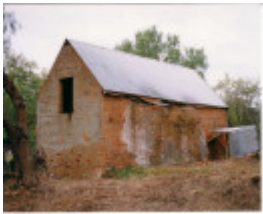
SM 17d - Stables building
