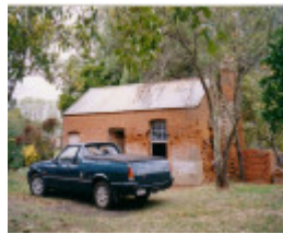
SM 17c - Kitchen building
