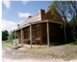
SM 17b - Store prior to renovation
