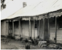
113391 B1694 Glynwylln Campbells Bridge nr Stawell
