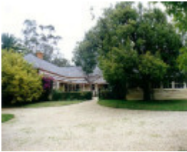
TO 01 - 'Tottington' Homestead and Outbuildings, Navarre Road, TOTTINGTON
