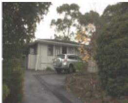
Front House June 2019
