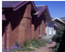
h00533 former police residence and lock up heales street talbot front corner she project 2003
