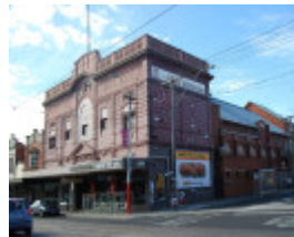
11447 Northcote Cinema 212 220 High Street View North East 31
