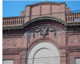
11447 Northcote Cinema 212 220 High Street Facade Detail 1 31
