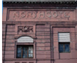
11447 Northcote Cinema 212 220 High Street Facade Detail 2 31
