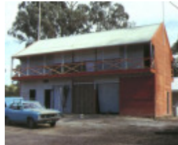
1 tarnagulla public reserve & cricket pavilion front view conserved grandstand
