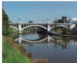
1 church street bridge from se bank mar01
