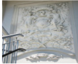
CHURCH STREET BRIDGE SOHE 2008
