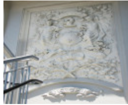
CHURCH STREET BRIDGE SOHE 2008
