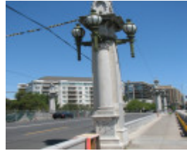
CHURCH STREET BRIDGE SOHE 2008
