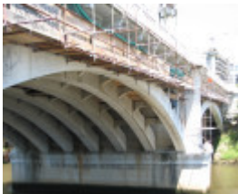
CHURCH STREET BRIDGE SOHE 2008
