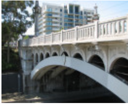
CHURCH STREET BRIDGE SOHE 2008
