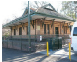
Yarra Park electrical substation July 2009
