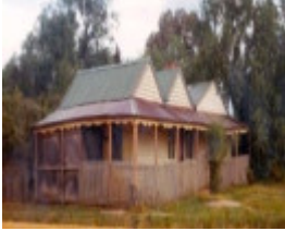
B3979 Fmr Butcher Shop & House
