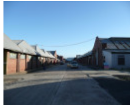
FORMER FEDERAL WOOLEN MILLS SOHE 2008
