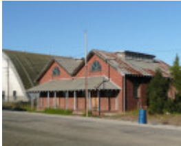
FORMER FEDERAL WOOLEN MILLS SOHE 2008
