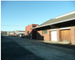
FORMER FEDERAL WOOLEN MILLS SOHE 2008
