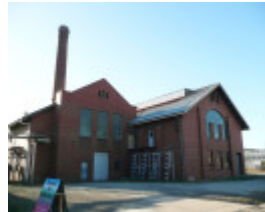
FORMER FEDERAL WOOLEN MILLS SOHE 2008
