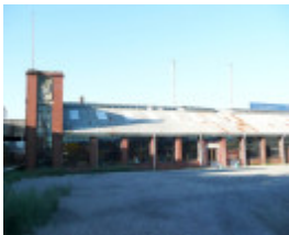
FORMER FEDERAL WOOLEN MILLS SOHE 2008
