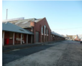
FORMER FEDERAL WOOLEN MILLS SOHE 2008
