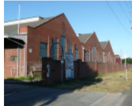
FORMER FEDERAL WOOLEN MILLS SOHE 2008
