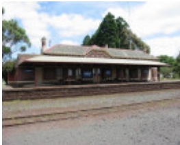
Terang RWS Station Building Platform February 2002
