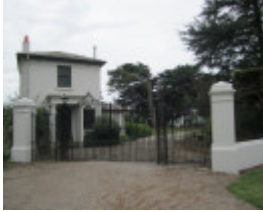
Front entrance showing Gatehouse
