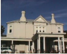
Cooring Yering House
