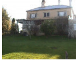
Cooring Yering House
