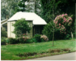
Dunbar Cottage and Dairy
