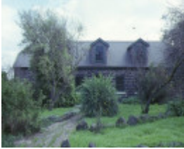
1 graffs farm thomas street thomastown front view
