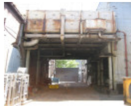
H2117 Overhead Water Tank Spencer St Power Station Rear View 6 Dec 2006 mz
