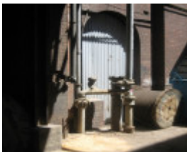
H2117 Overhead Water Tank Spencer St Power Station Associated Pipework 6 Dec 2006 mz
