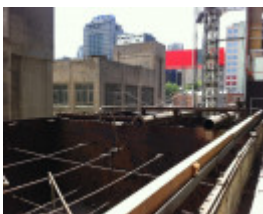
Internal tie rods
