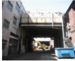
H2117 Overhead Water Tank Spencer St Power Station Front View 6 Dec 2006 mz
