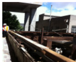
remedial works commence Nov 2011
