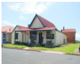
TINTALDRA GENERAL STORE AND FORMER BAKERY SOHE 2008
