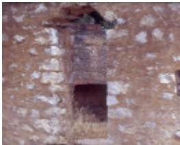
h01959 stasinowskys lime kiln chain road pella doorway she project 2004
