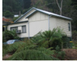
rear of building
