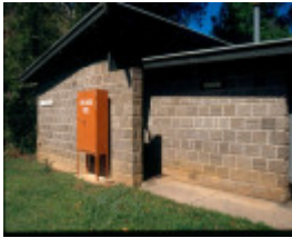
Spring Creek Toilet
