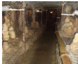
Typical netting inside caves. May 2007.
