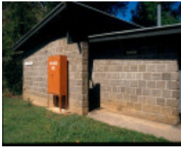
Spring Creek Toilet
